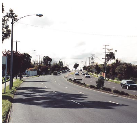
Removal of the centre lighting poles has made the road safer.
