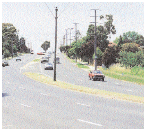
Non-frangible light poles, especially in exposed places close to the carriageway on a bend, are a definite road hazard.
