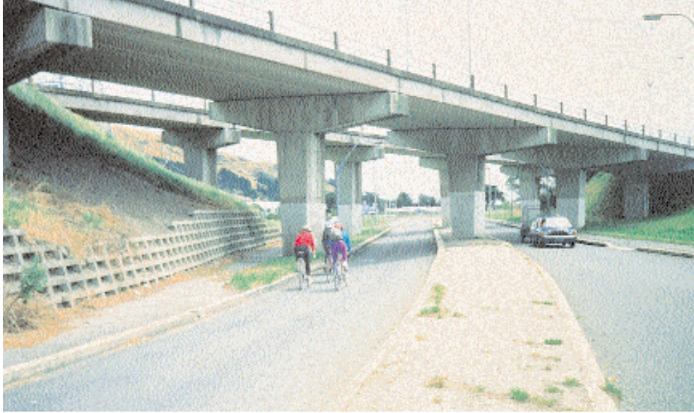
Bridge piers restrict forward sight distance at the location proposed for a new right turn.
