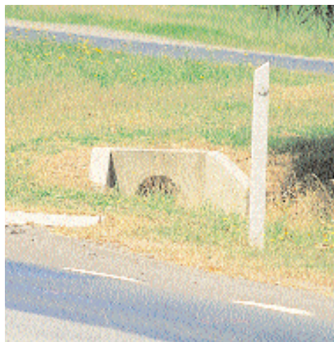
End walls of culverts, if near roads, can be replaced with covered drains, or with angled end walls, or shielded with crash barriers.
