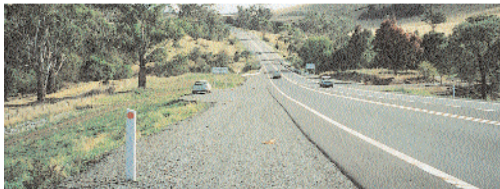
After audit, the delineation and crash barriers have helped to minimise accident risk at this site, pending future widening.
