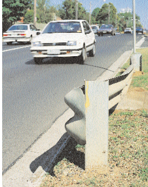
Crash barriers need to be sufficiently long in order to have adequate strength. The ends should not be a hazard, and the barrier should be anchored and otherwise installed in accord with standards.
