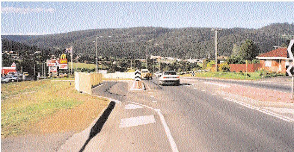
A driveway into a fast-food development has been designed with safety in mind: fencing is installed to prevent pedestrians crossing where it is dangerous. But the island for the fencing results in a tight exit off the road and the fencing is very likely to be struck by errant vehicles.
