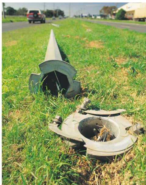
Non-frangible light poles, especially in exposed places close to the carriageway on a bend, are a definite road hazard.
