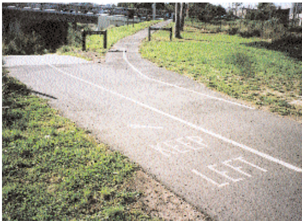
The link path from Toorak Road joins at an acute angle, with restricted sight distance.
