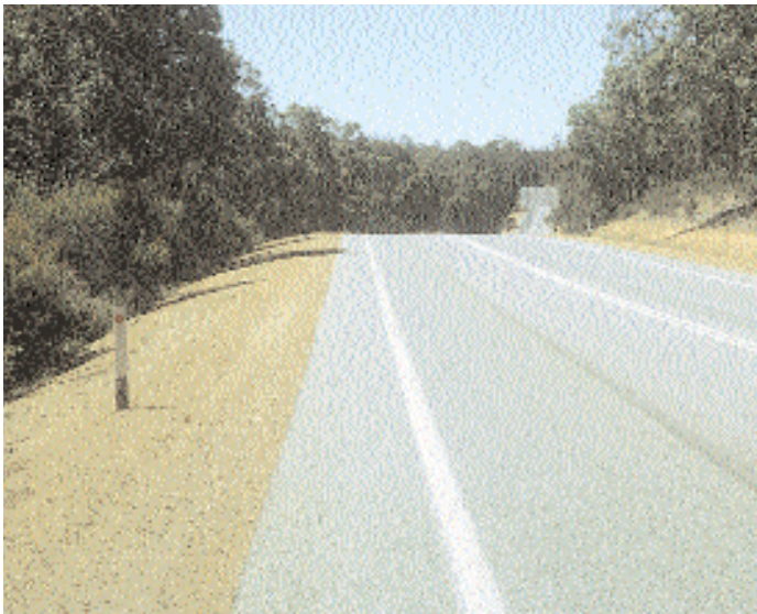
A summit vertical curve restricts the driver's view of the start of the horizontal curve and may produce a dangerous situation.
