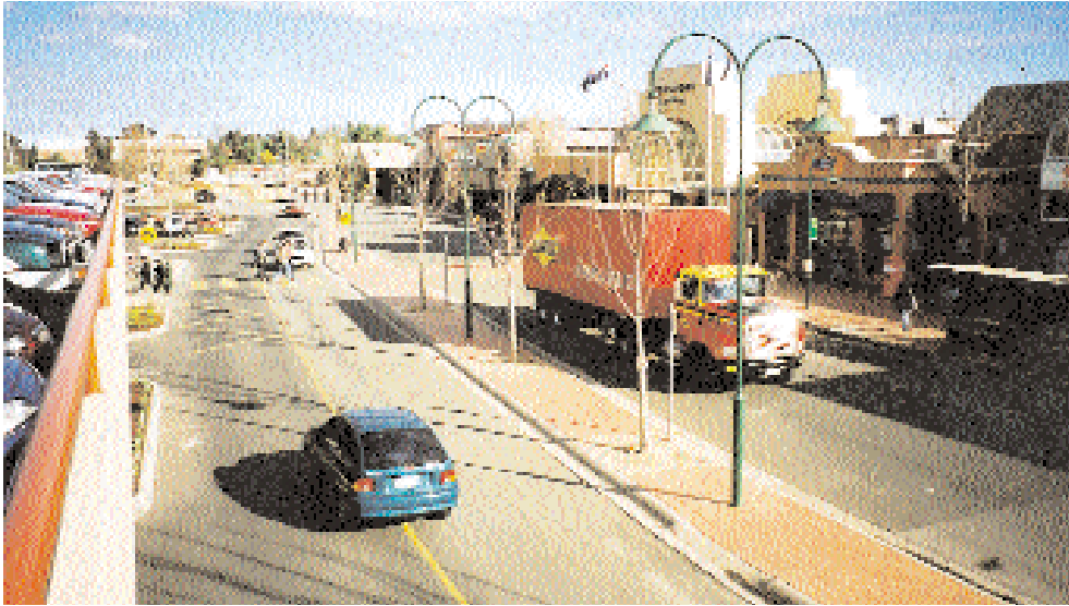
This two-way road (left) and one-way service road (right) at a shopping centre can easily be mistaken for a divided road, with serious consequences for pedestrians.
